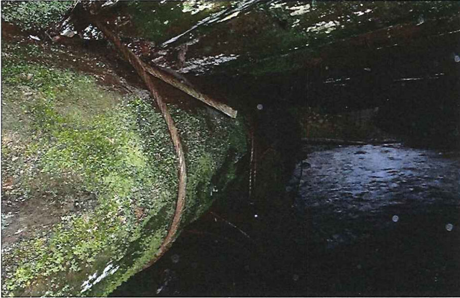
CK2346 Left Abutment
